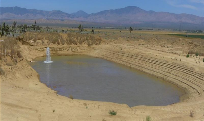
Infiltration from ponds
